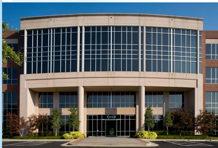
HCA Center for Clinical Advancement at The Boulders 7300 Beaufont Springs Drive BLDG VIII, Richmond VA
